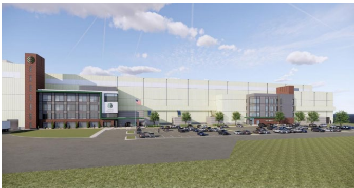
Figure 16 – New CRB mill, consolidating 4 mills into 1
